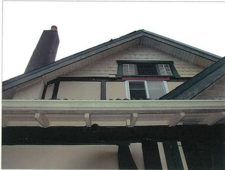
Exterior Gable End & Chimney
